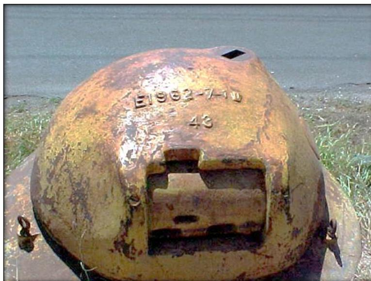
Photo shows the closed firing embrasure of an example found outside the security fence at the former Lualualei NRS. (Photo by author)
